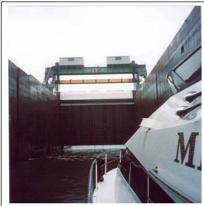
Lock 17. Gate is opening on the largest vertical door lock in the world.
